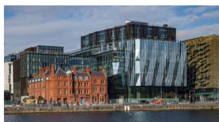
Adare Office Asset – Dublin, Ireland
